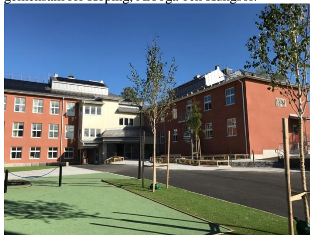
S:t Olovsskolans annex, renoverat under 2016/17
