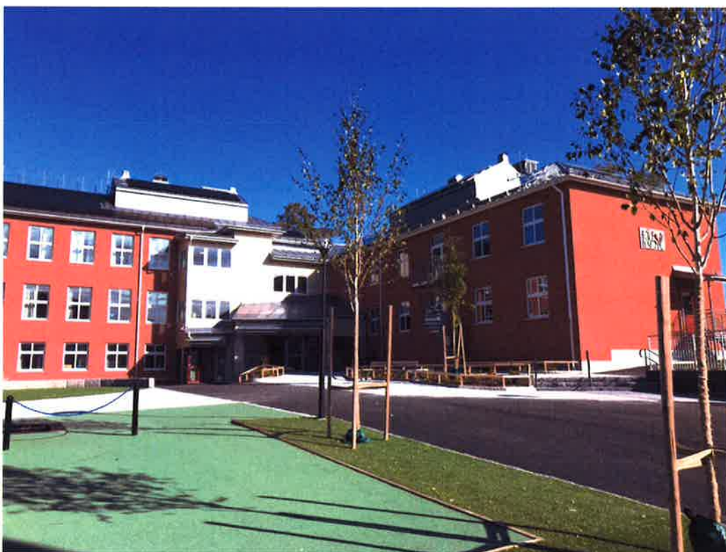
S:t Olovsskolans annex, renoverat under 2016/17.
